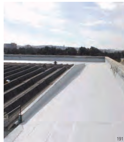
Industrial rooftop applications.
