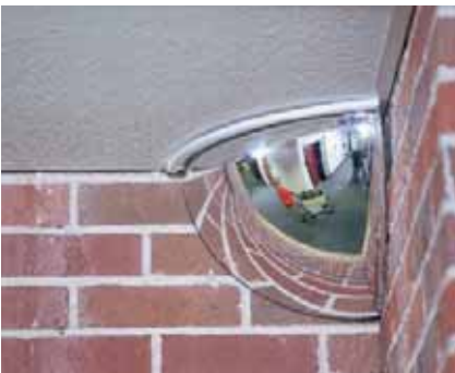
Dome - prevents collision in high hazard areas.
