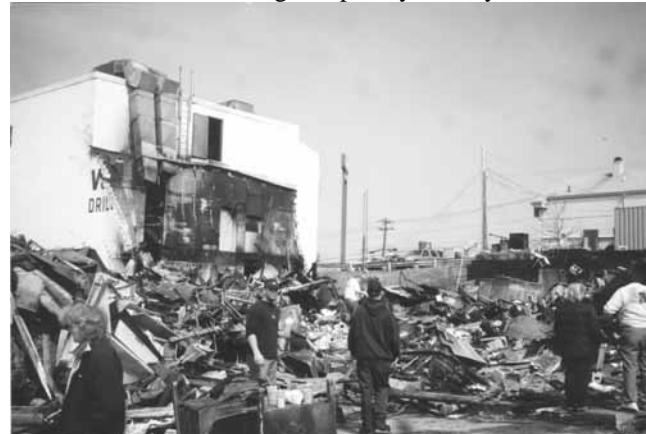
Front and side of building completely destroyed.
