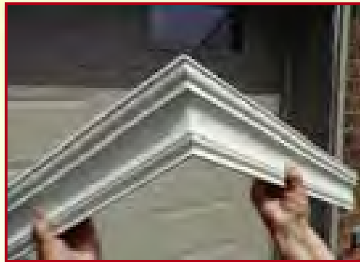
Create perfectly fitting exterior crown molding joints
