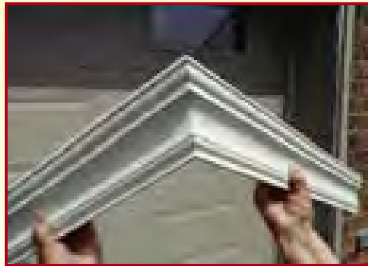
Create perfectly fitting exterior crown molding joints
