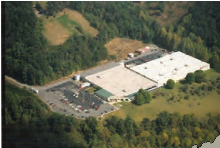
Our 168,000 ft 2 facility in Murphy, North Carolina employs 300 associates. Each tool is designed and manufactured right here, with a distribution center that ships daily around the globe.
