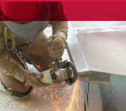
Grinding on a platform for weld preparation.
