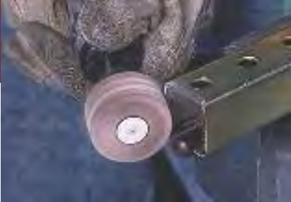
Deburring perforated steel channel after saw-cut.
