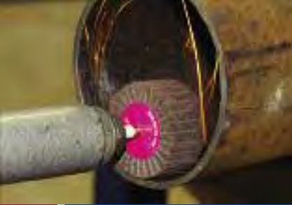
Deburring the I.D. of a steel pipe with an interleaf flap wheel.
