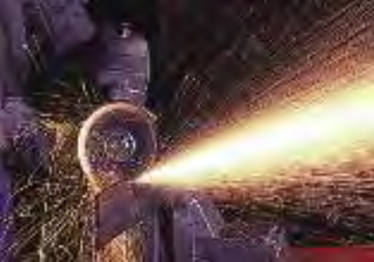
Notching a steel bar prior to welding.
