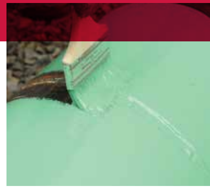
Applying pipe coating to weld seams.
