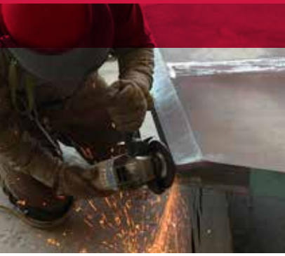
Grinding on a platform for weld preparation.
