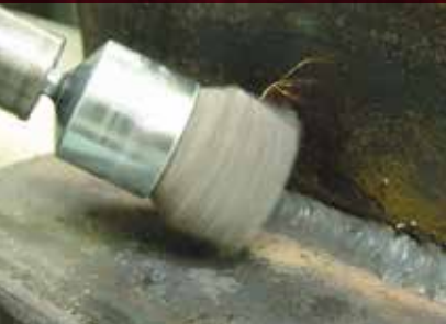
Cleaning hard-to-reach fillet welds with a Controlled Flare End Brush.
