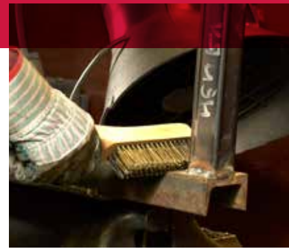
Cleaning surface rust in order to repair a weld.
